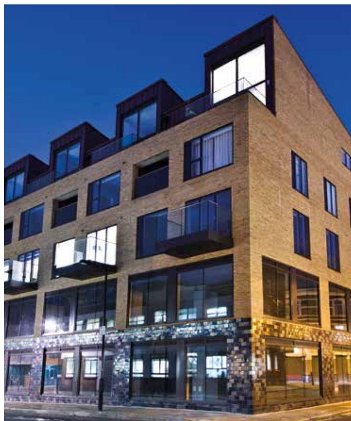
Newspaper House, Rushworth Street SE1
