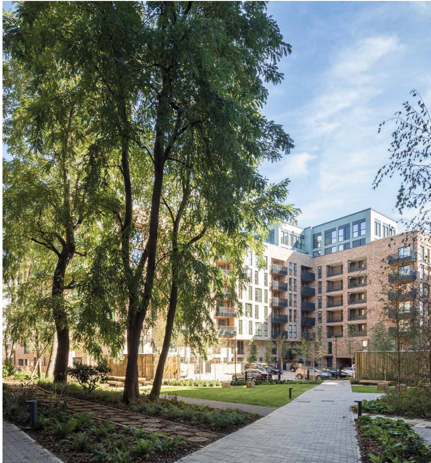
Photography of one of the completed phases at Acton Gardens.
