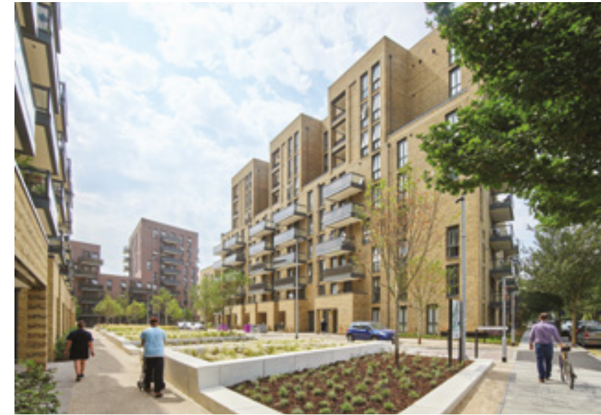
ST PAUL'S SQUARE, TOWER HAMLETS, LONDON ▲
