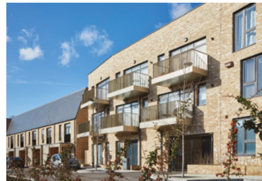
BROOK VALLEY GARDENS, CHIPPING BARNET, LONDON ▼
