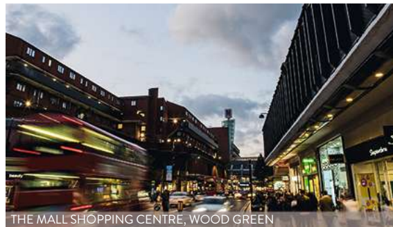
THE MALL SHOPPING CENTRE, WOOD GREEN
