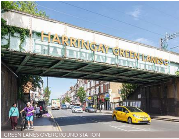
GREEN LANES OVERGROUND STATION
