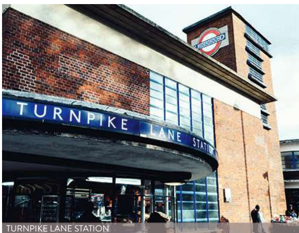
TURNPIKE LANE STATION
