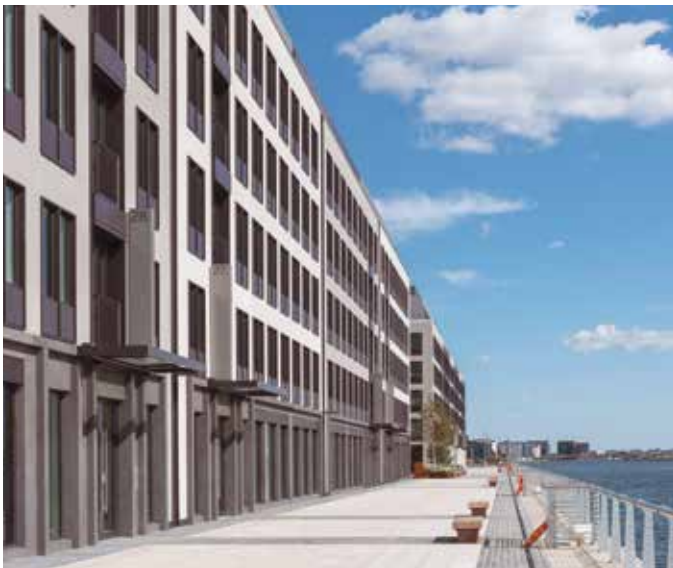
BRUNEL STREET WORKS
