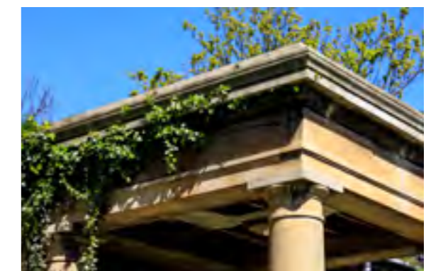
Corner detail on the entrance portico at the historic Chapel building, built in 1928 - 1929 to commemorate Miss Richardson, a former lecturer at Westfield College
