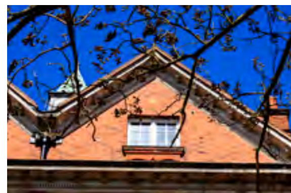
The red-bricked gable of Chapman supports a proud cornice with detail brackets from Roman cement
