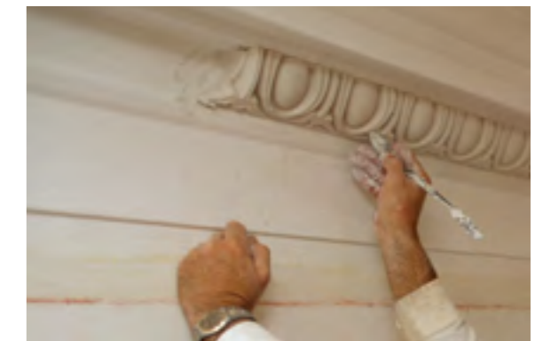
An architectural restorer carefully reworks carved plaster Ionic 'egg and dart' detailing
