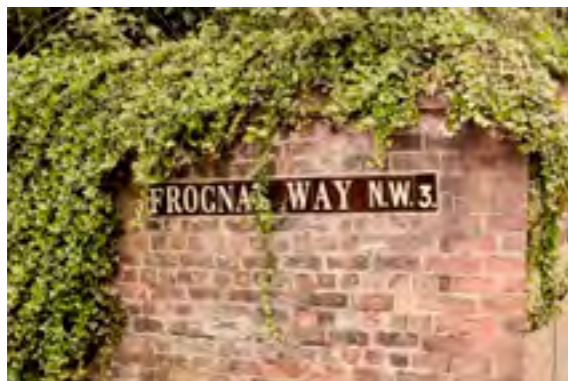
The signature soft red brickwork of Hampstead
