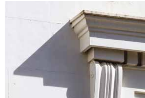
White stuccoed entablature detail on Kidderpore Hall
