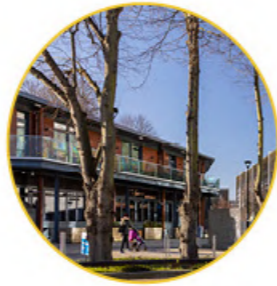
HIGHAMS PARK TOWN CENTRE
