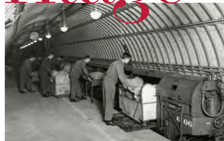
23 miles of underground railway were used to deliver post around London
