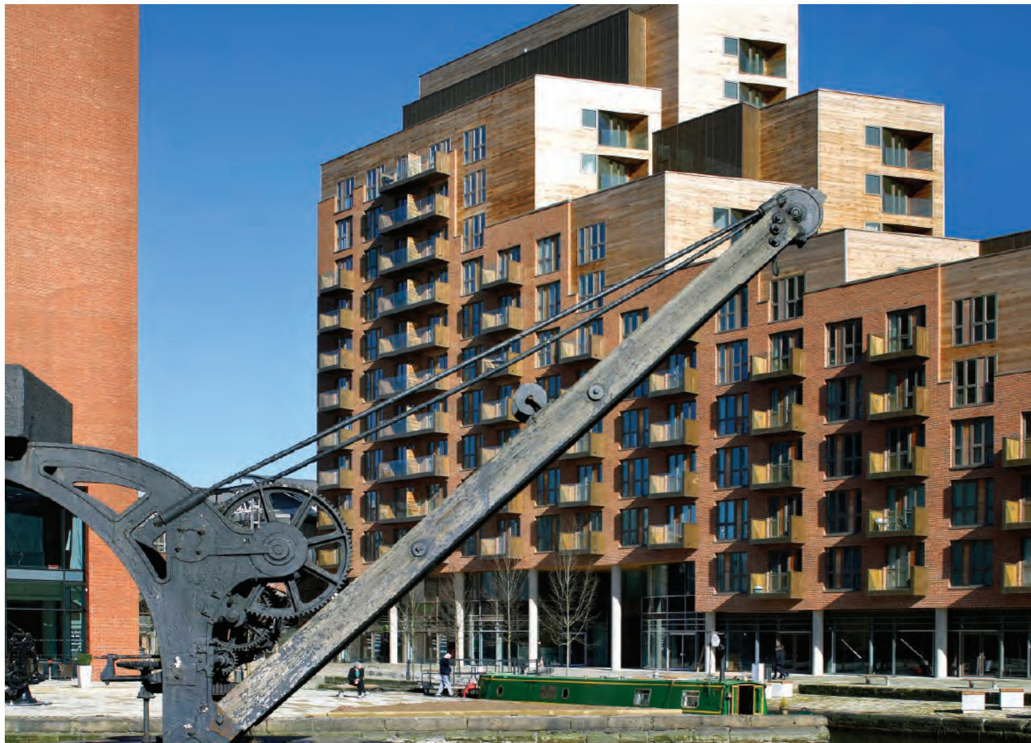
IMAGES OF BRENTFORD LOCK WEST AND GRANARY WHARF, WATERSIDE PLACES
